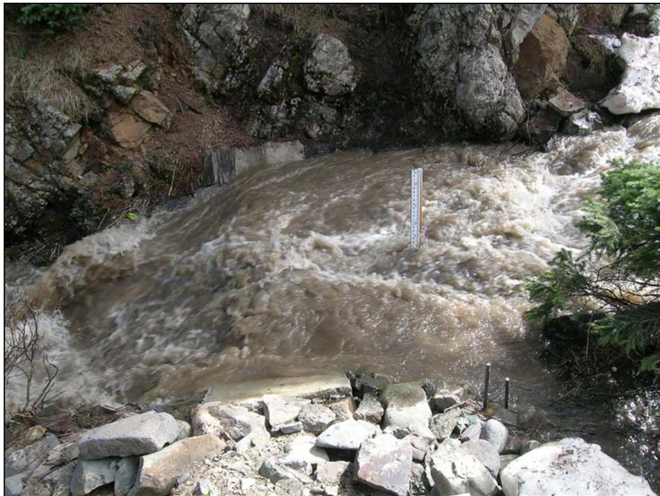
*Figure 3: the Senator Beck Basin broad-crested weir just hours before 2010 peak flow on June 5, 2010.*
